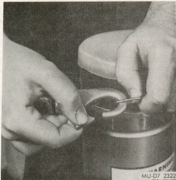
Figure 3-9. Static line attached to lanyard.
