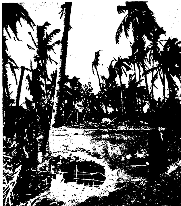
Figure 109. Concrete pillbox on Guam.
