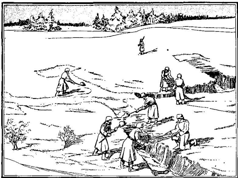
Figure 64.—Camouflaging trenches with willow frames.
