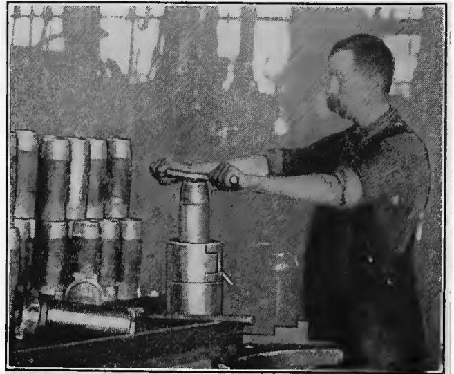
FIG. 14. FITTING DRIVING DOGS AND CENTER PLUGS FOR GRINDING
