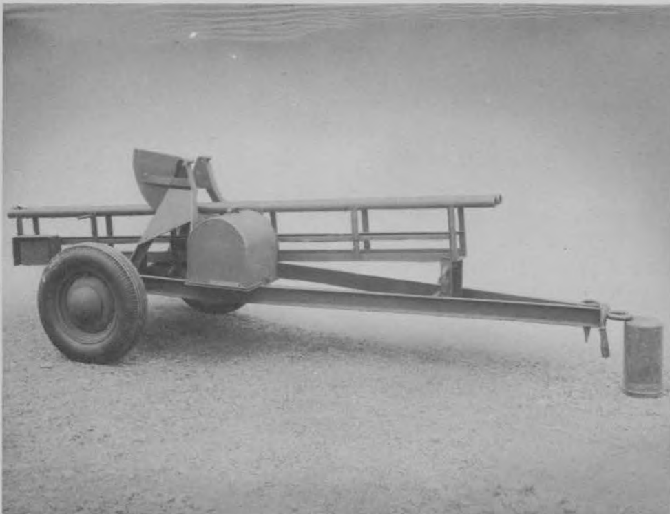
ROCKET TARGET PROJECTOR, M1, IN TRAVELING POSITION
