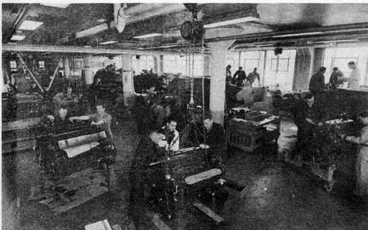
Students assembling engines and installing them in tank hulls at the Detroit Diesel Engine Division's Tank School held at General Motors Institute, Flint, Michigan
