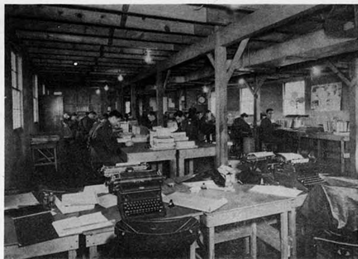
Instructors' Office, Supply and Military Administration Section
