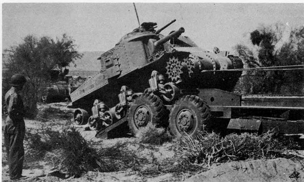
Showing skid in place to guide tank onto trailer while being loaded
