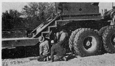
Preparing to drop the T-3 trailer
