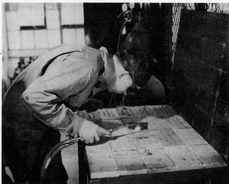
Figure 9 -- Oxyacetylene welding on M3 welding truck
