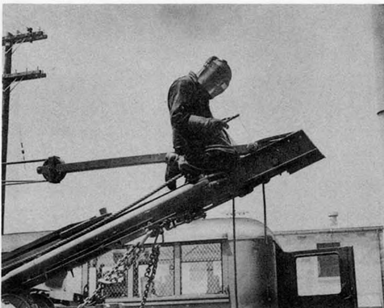
Figure 23 -- Field repair of boom on M1 wrecker by arc welding, using M3 welding truck
