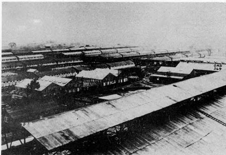
Section of World War powder plant used as a post war "dump" for 52,000,000 pounds of smokeless powder, stored in metal lined wooden boxes. Storage classed as "temporary".
