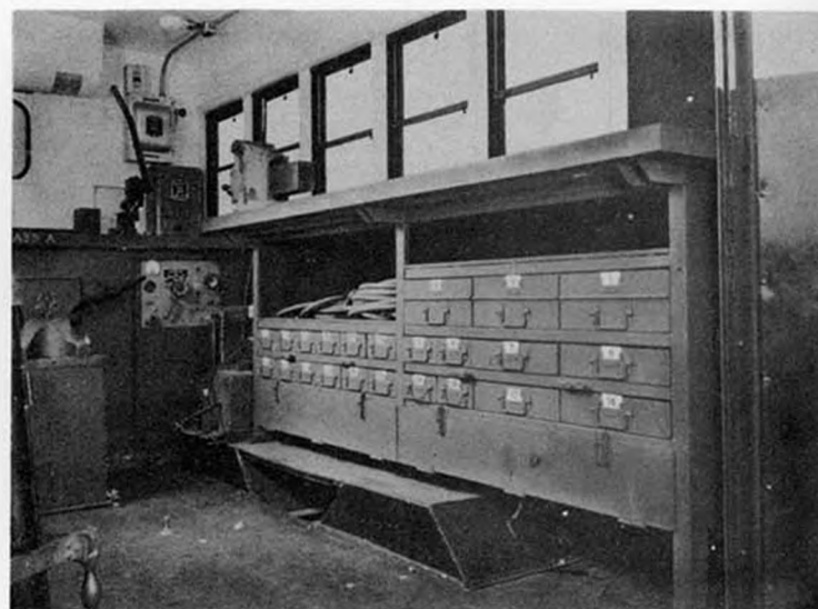
Figure 31 -- Work bench and electrical controls, welding truck M12
