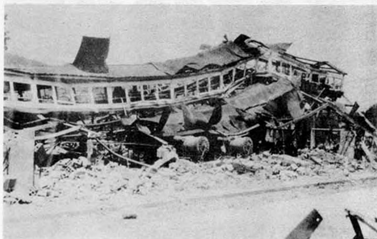
Effect of explosion on hollow tile and wood construction. Building was 1250 feet away.
