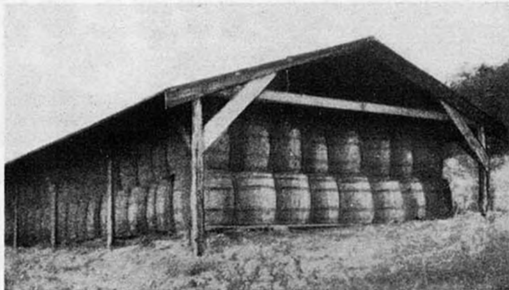
"Temporary" post war magazine holding 200,000 pounds of dry picric acid in wooden barrels, holding 400 pounds each.
