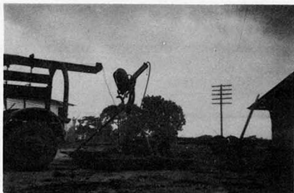
The platform "in position". Spurs are provided for assurance against shifting while on the trailer, and they also prove useful as "spikes" when platform is on its ground position.
