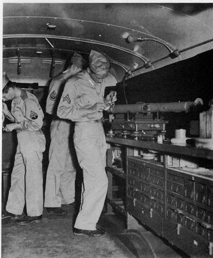
Fig. 4 -- With blackout curtains in place the maintenance operations are limited to those involving no use of outside targets. Above: instrument repairman working on a range finder, with blackout curtains in place.
