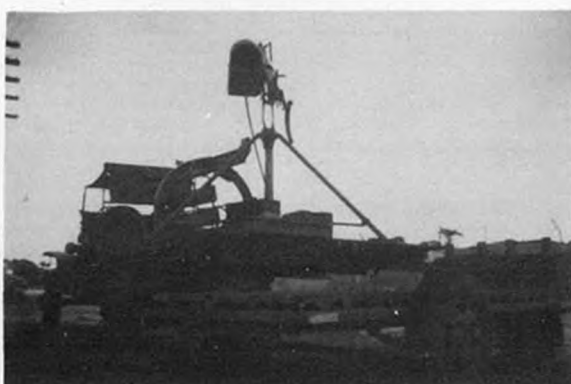
Bomb truck lifting trailer. The cable is hooked on the mount at the turnbuckle.
