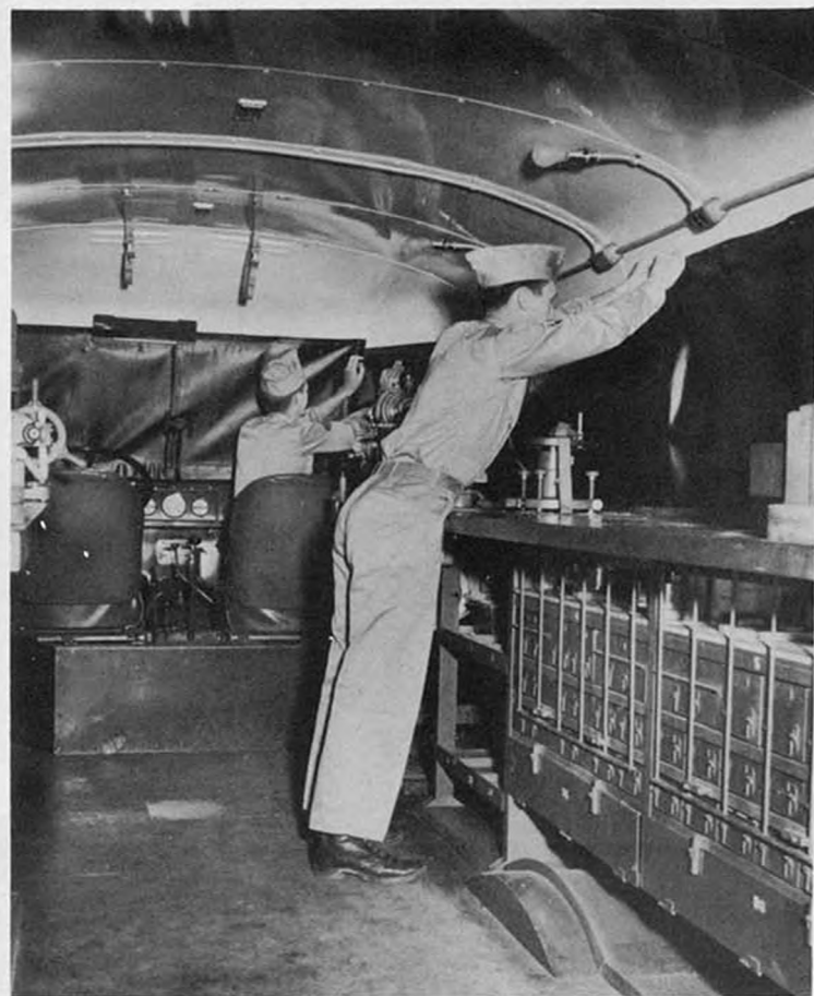
Fig. 3 -- Blackout curtain, shown being adjusted above, are an integral part of the equipment of the Instrument Repair Truck.
