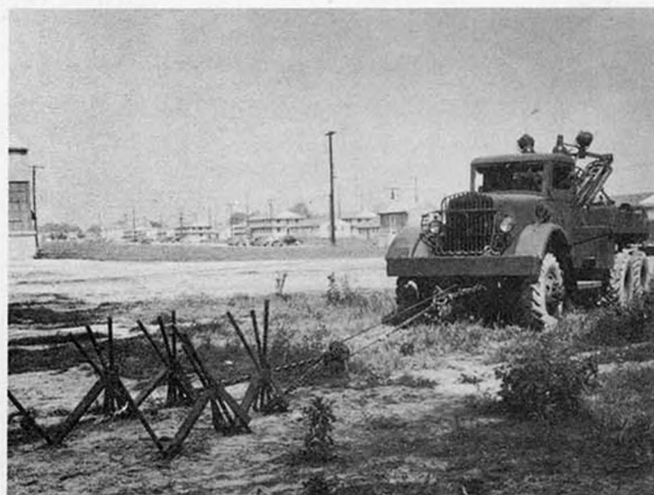
Figure 2 Wrecker anchored in front for rear recovery operations.
