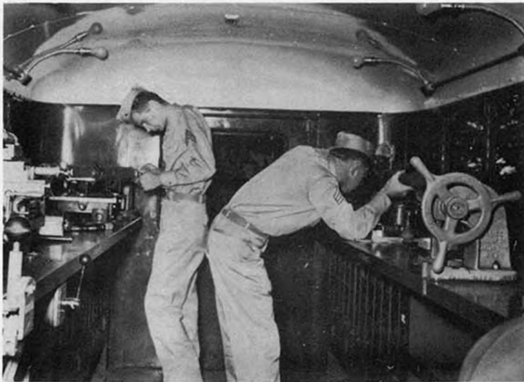
Fig. 9 -- When it is not necessary to use blackout curtains, instruments may be adjusted inside the truck. Even at night adjustment is possible. The moon and stars furnish excellent targets for "infinity" adjustments.
