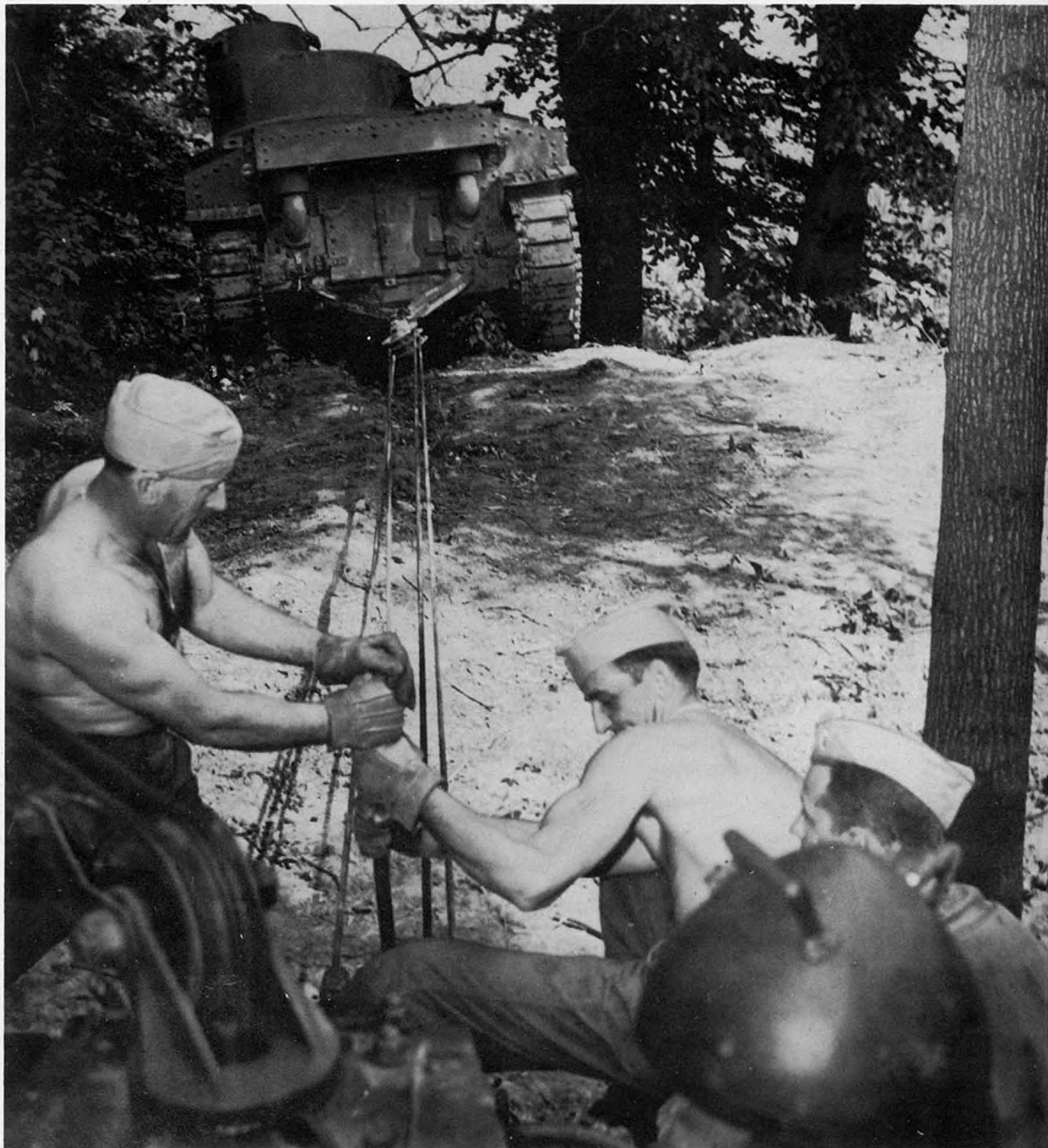
Figure 14 Tank at top of grade . . . .
