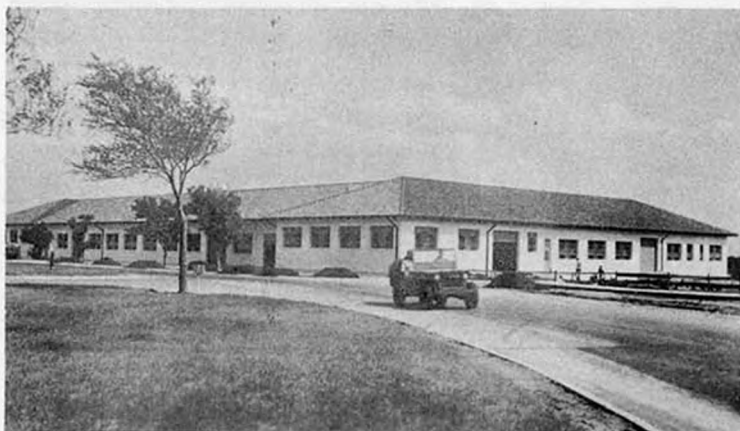
Recently completed building housing the Materiel Department. Field Artillery School, Fort Sill, Oklahoma
