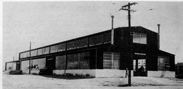
One of the recently completed units in the Ordnance Area, Fort Sill, Oklahoma
