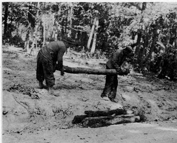
Placing logs in a ditch to give an additional inlet to an Ammunition Depot.
