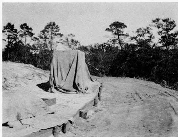
A section of the Magazine Area, showing clay road on sand adjacent to the tarpaulin-covered bombs. Layout facilitates one-way traffic and easy access to materiel. A new and much larger Magazine Area is now under construction and will be one of the largest and most modern in the Southeast Air Corps Training Center.
