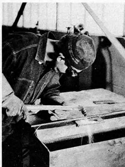
Plate beveling with a manually operated cutting torch
