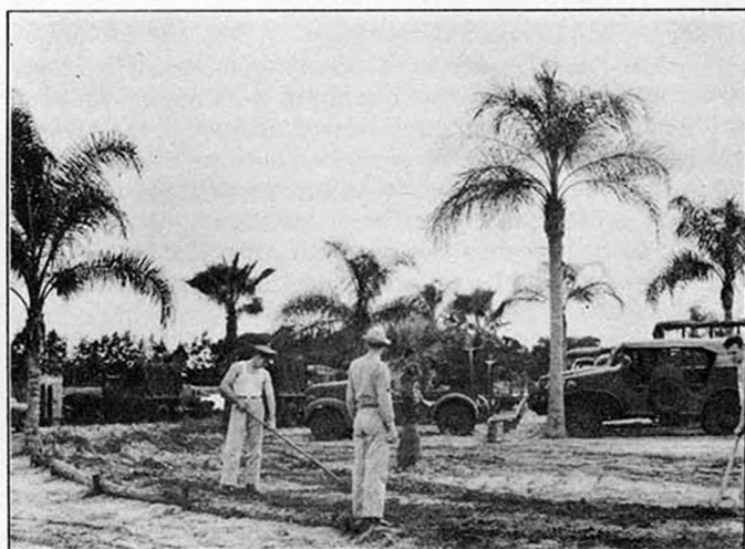
Making a clay road into our SANDY motor pool. It helps.
