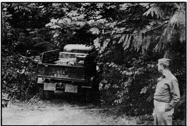
Ammunition carrier entering Ammunition Depot
