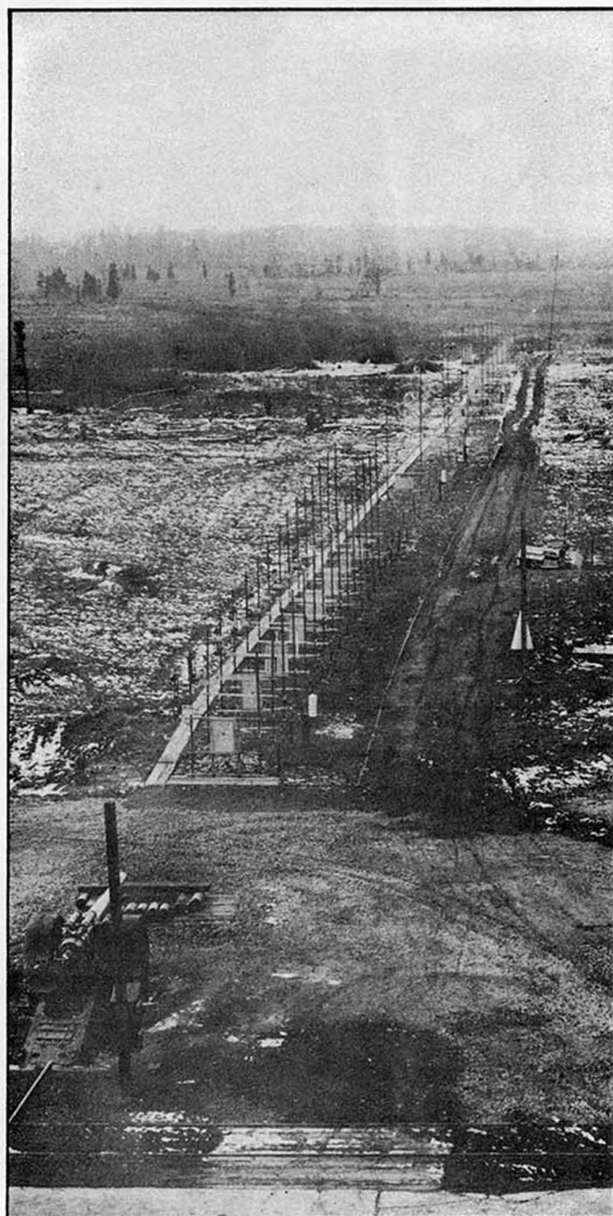
Figure 3 Exterior of ballistics firing range.
