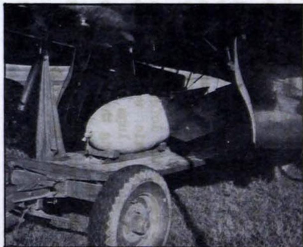
1100 LB. BEING SECURED IN THE BOMB BAY OF A LARGE ARMY BOMBER.
