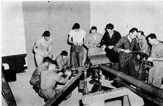
Detailed disassembly of the 75 mm Gun and Carriage, M2A2.
