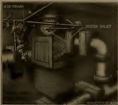
Fig. 7.—Pyro Discharge to Boiling Tubs (1st Floor).
