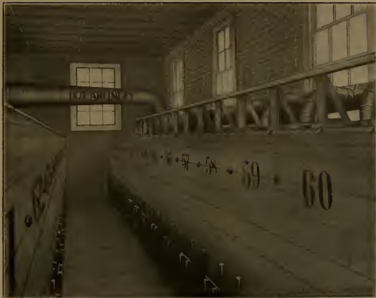
Fig. 23.—Typical Interior of Dry House.
