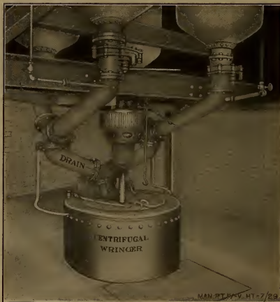
Fig. 6.—Nitrating House (2nd Floor).
