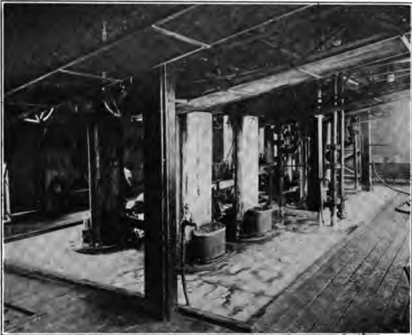
PLATE 1.—DU PONT MECHANICAL DIPPER PROCESS, NITRATING FLOOR, SMOKE- LESS POWDER FACTORY, PICATINNY ARSENAL, N. J.
