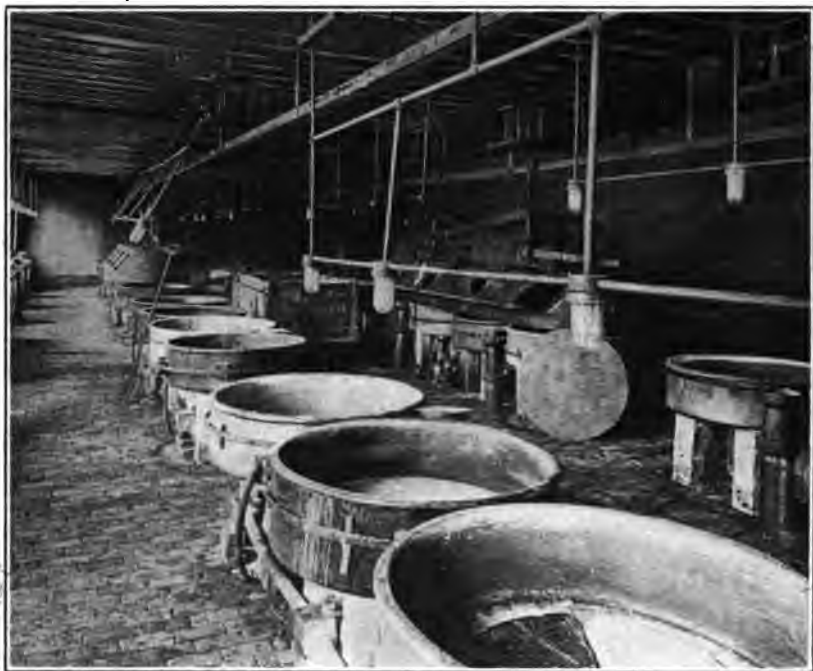
PLATE 4.—NITRATING PANS, THOMPSON DISPLACEMENT PROCESS, SMOKELESS POWDER FACTORY, PICATINNY ARSENAL, N. J.
