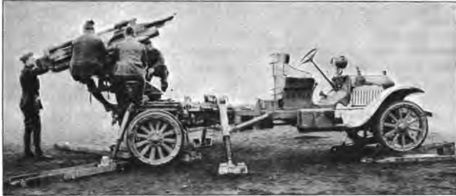
VIEW SHOWING TRUCK MOUNT IN ACTION.
