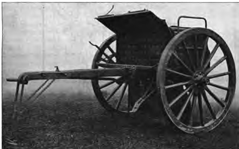
FRONT VIEW, SHOWING DOOR SWUNG UPWARD EXPOSING AMMUNITION.
