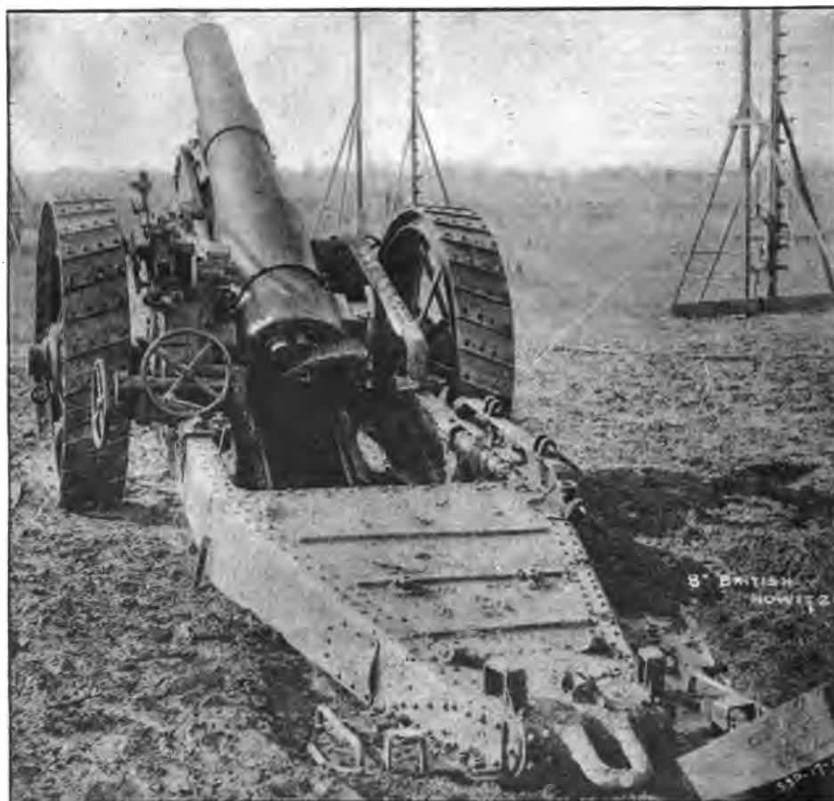
REAR VIEW OF CARRIAGE, SHOWING MAXIMUM ELEVATION OF HOWITZER.
