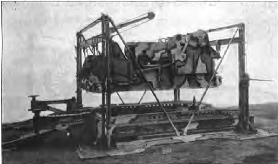
LOWERING THE TOP CARRIAGE IN POSITION.
