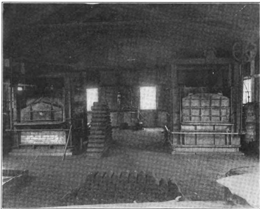
FIG. 392. HEAT TREATING DEPARTMENT
