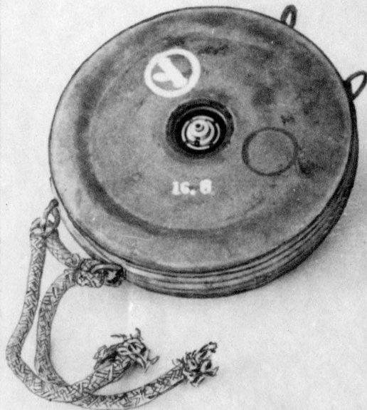
JAPANESE ANTI-TANK MINE TYPE '93. ( TYPICAL PACKING )
