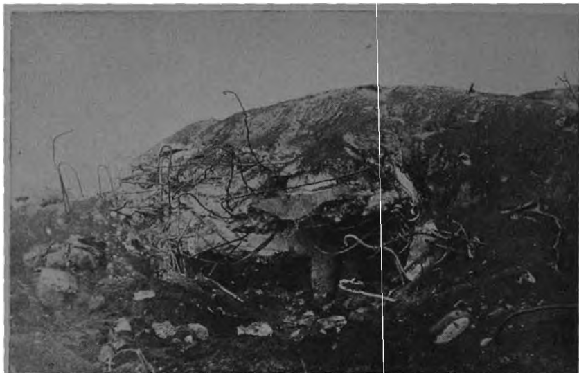
Many pillboxes were made of steel-reinforced concrete, some as much as 4 feet thick. This one, which housed a 25-mm automatic cannon, overlooked Red Beach Number One.
