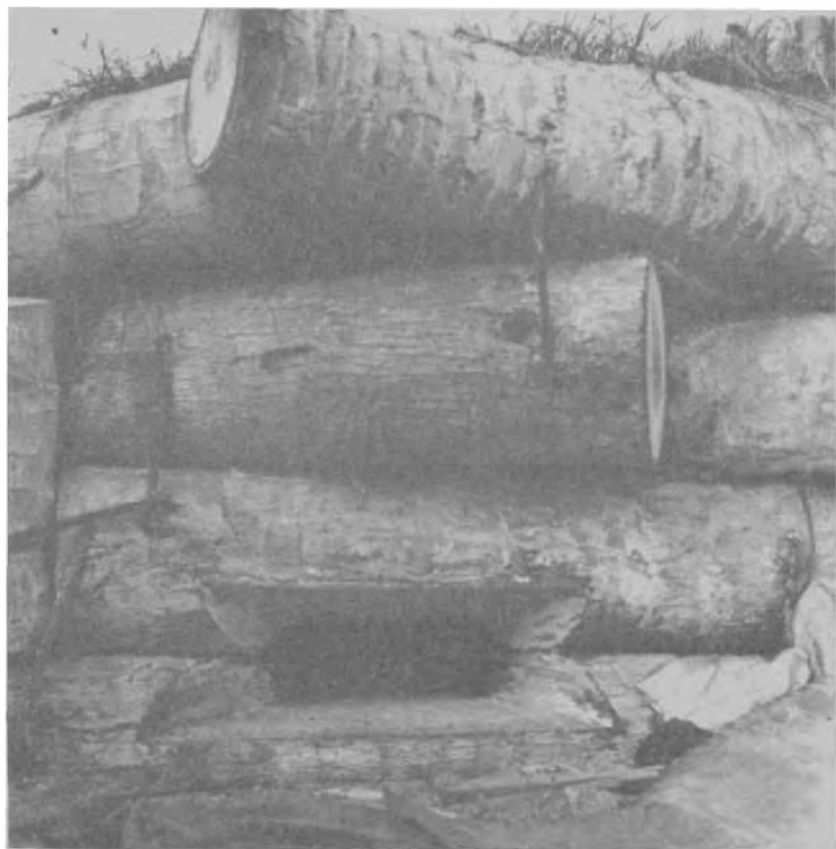
Figure 4.—Front View of Typical Japanese Pillbox (Betio).
