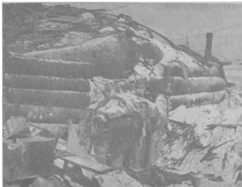
Figure 12.—Japanese Shelter (Betio).
