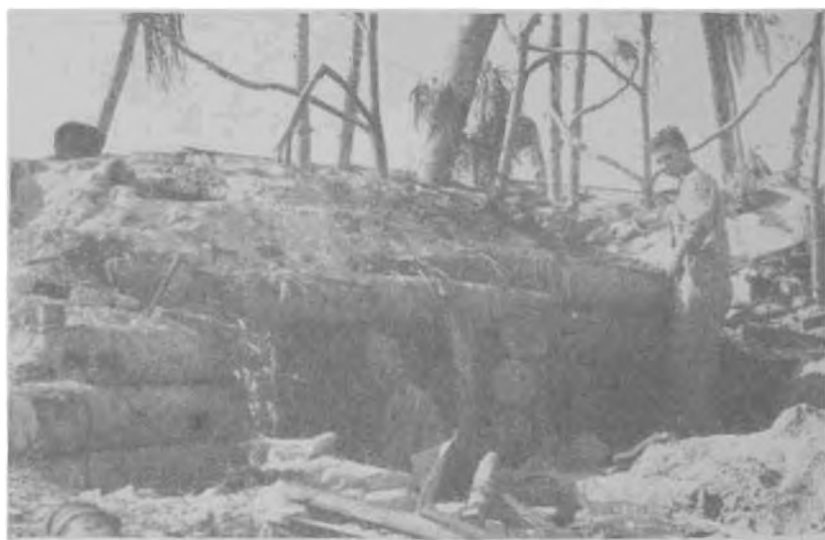
Figure 11.—Japanese shelter (Betio).
