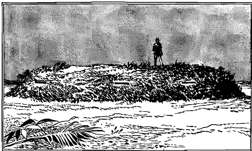
Figure 3.—Typical Japanese Bunker.
