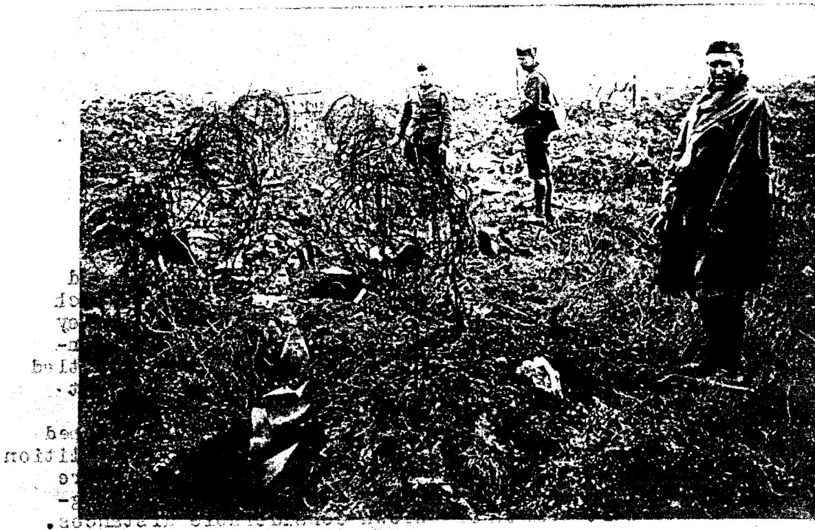
Showing the manner in which mine fields were camouflaged and protected with barbed wire and barbed wire concertinas.
