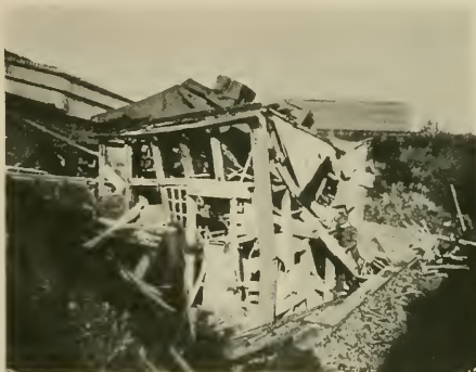
FIG. 139. Building wrecked by Explosion 30 yards away. Ardeer, February 27, 1897
