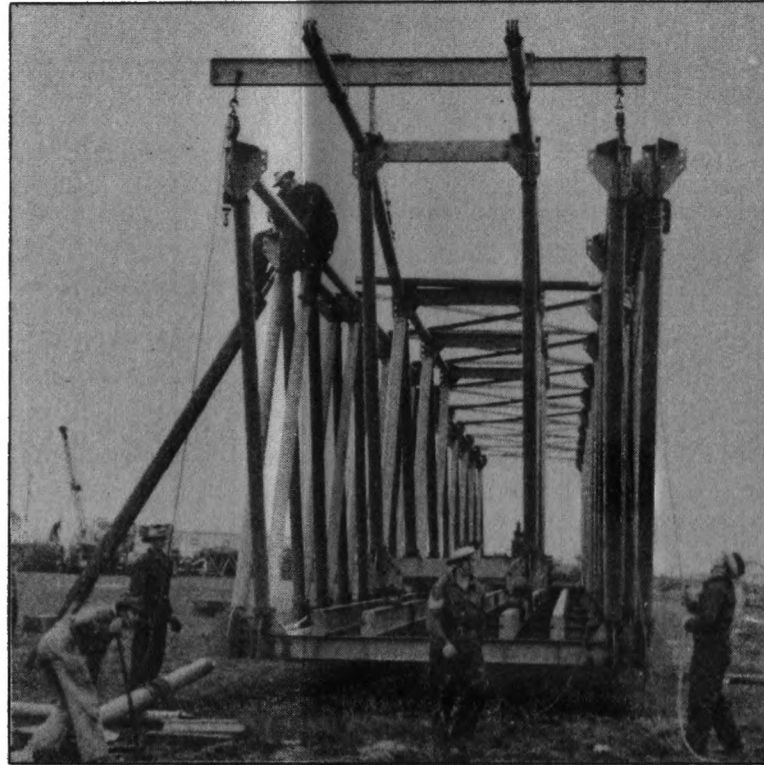
No. 2 ERECTION TROLLEY - EXT.
