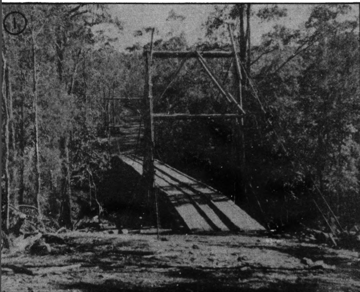
View of Bridge
