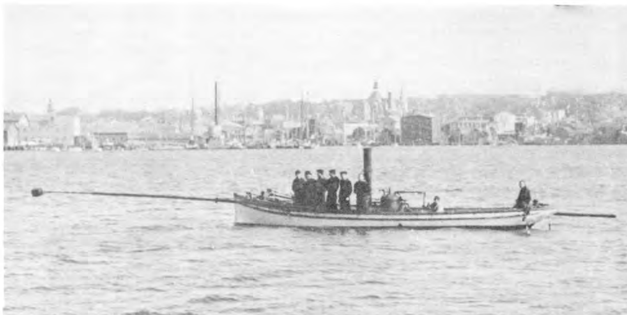
Figure 2. Spar Torpedo Rigged for Test from Bow of Steam Launch
